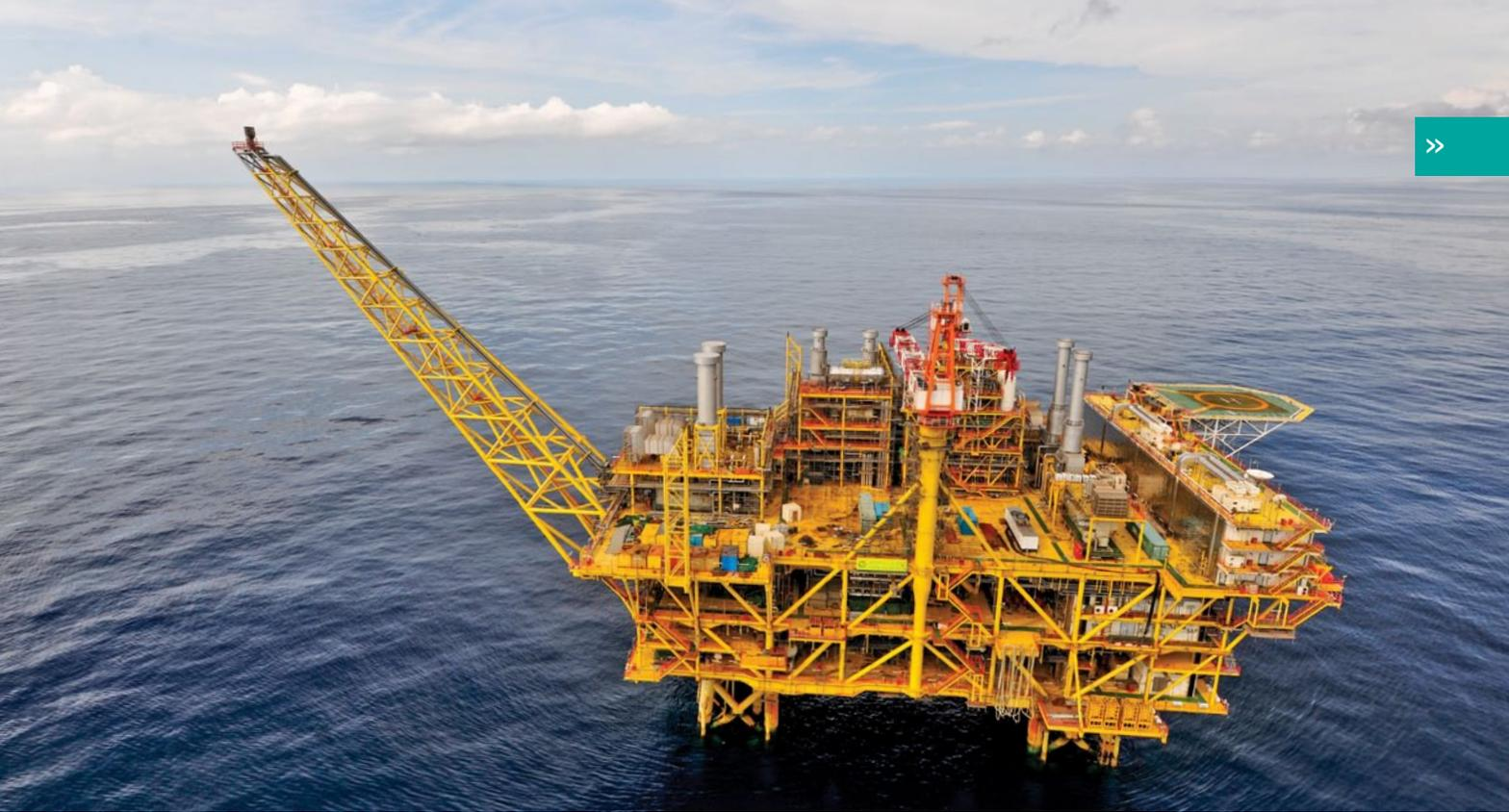
pipes to the onshore processing plant in Zhuhai. Engineers claim this is economic as a single platform can process the output from several nearby oil/gas fields, reducing the amount of deep-sea piping needed to transport output to the onshore gas processing plant.
